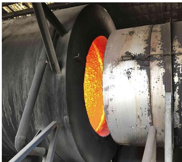
Image 3. EPA 2 – Cooling Air Vent
