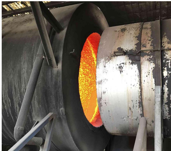
EPA 2 – Cooling Air Vent
